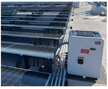
The project's total size is 331 kW with an estimated annual production of 450,000 kWh. This production offsets 70% of the energy needs for the facility. This array features 566 Trina solar panels and 5 SMA CORE1 inverters. SMA and racking manufacturer Sollega engineered the first solution commissioned in New Jersey that meets the UL 3741 certification, together with Equinox Renewable Energy.
